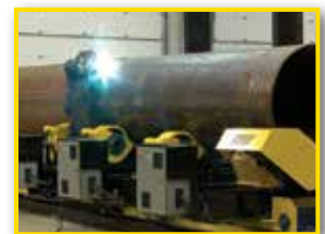
Ready for fit up and/or automated welding, then index for next section to be added.
